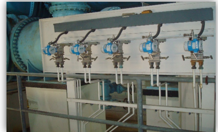
Bank of Differential Pressure Cells connected to flowmeters (Courtesy of Louisville Water Company)
