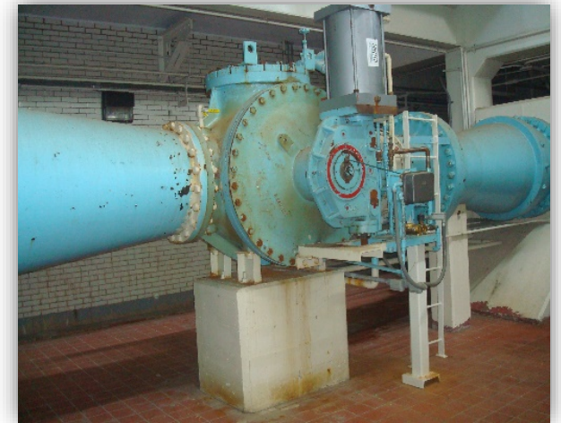
Venturi meter with valve in the throat
