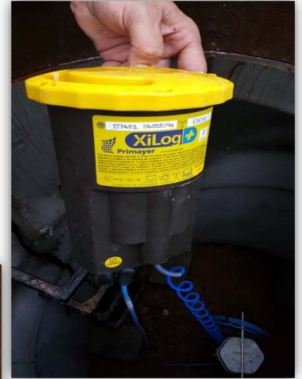
Primayer Xilog data logger records data on site
