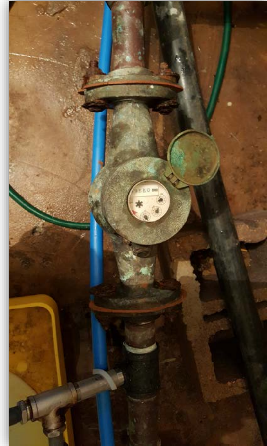
Old 1.5-inch turbine meter measuring treated water from a well in a system serving 1,100 people
