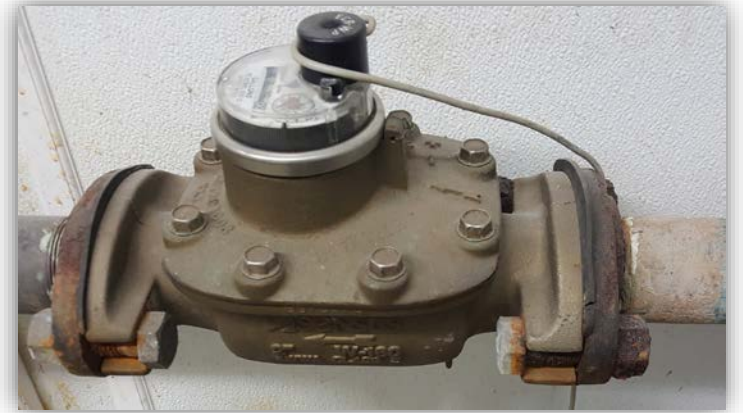
Full-bore 2-inch positive displacement meter
