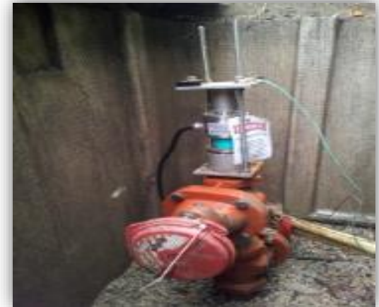
Insertion magnetic flowmeter on a 30-inch pipeline
