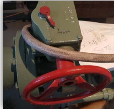
Mostly closed butterfly valve next to a flowmeter used to control flow to 144 gpm, but serves as an obstruction
