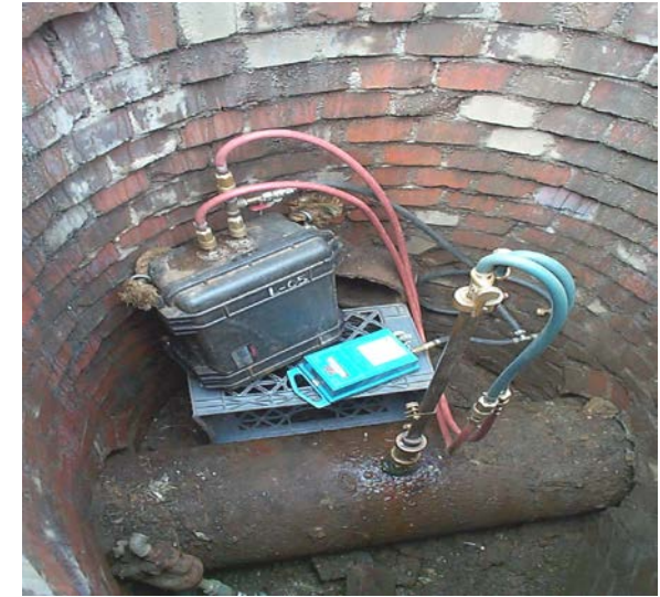
Pitot rod inserted in a 12-inch pipeline
