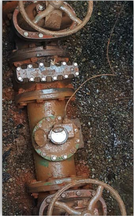
8-inch turbine meter measuring flow to a system serving 1,000 people
