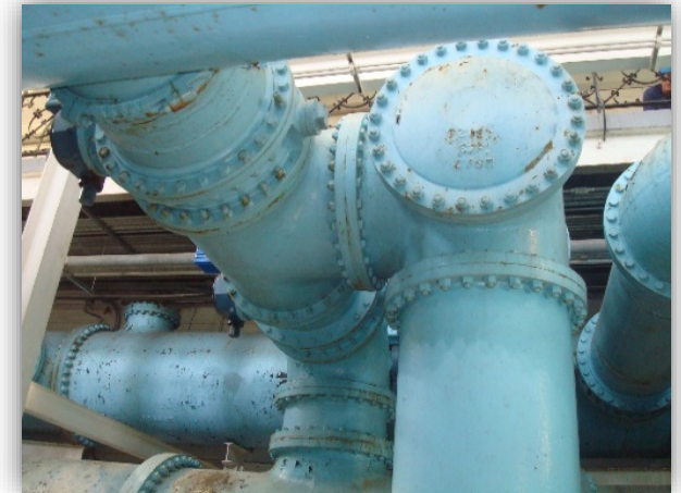
Maze of pipe bends downstream of the above flowmeter
