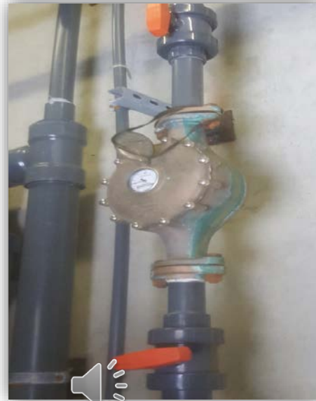
6-inch turbine meter installed in the vertical position
