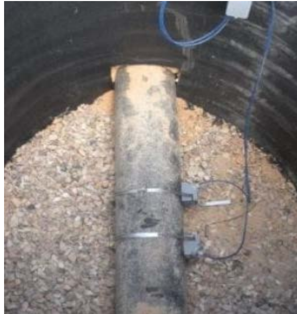
Strap-on ultrasonic flowmeter installed permanently Source: Frontier Precision
