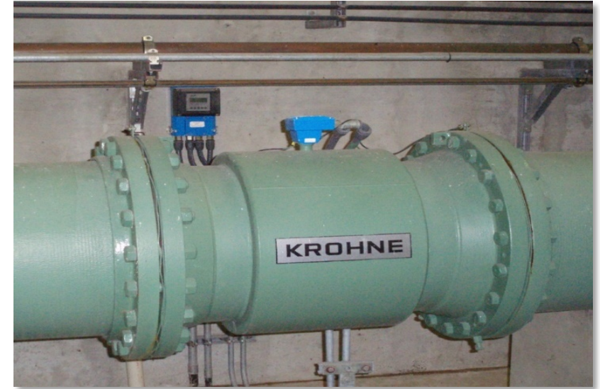
A "magmeter" measuring flow leaving a water treatment plant
