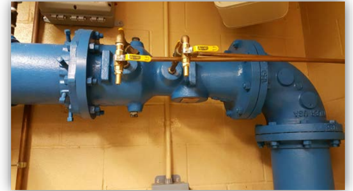
12-inch venturi flowmeter measuring imported water
